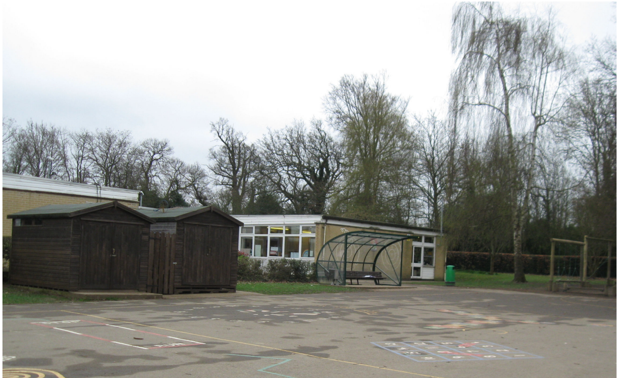
Photograph of the site showing the two sheds to the west and the shelter to be relocated
